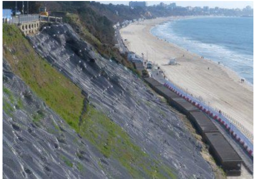
Photo: Cliff erosion protection scheme 2021
